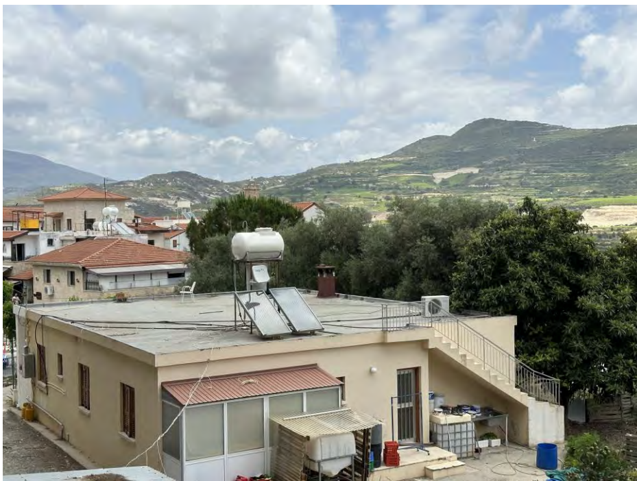
Solar water heater on top of the houses. Sunshine most of
