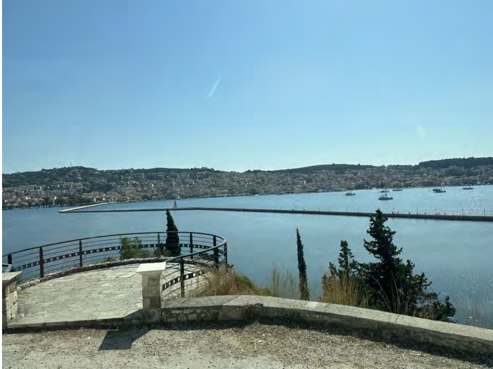
Overview of the bridge. Used only for pedestrians now.
